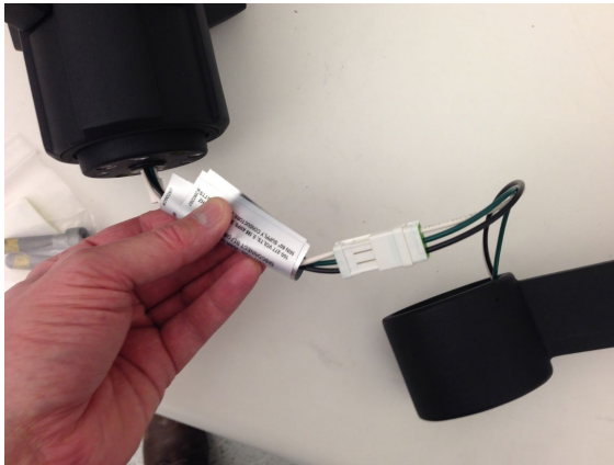
Fig. 2– Wall mount luminaire to bracket wiring connection
